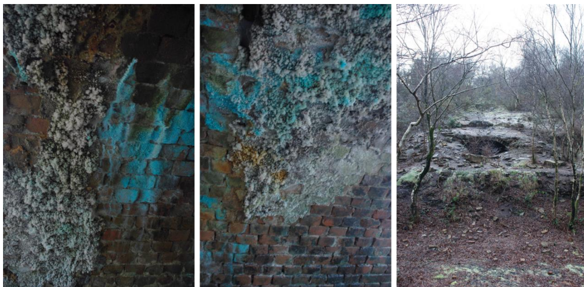
Figure 3-5 Image across the top of the row of calciners at New Great Consols (right, east to west) and the efflorescent precipitates on the inside of the structures, with typical whitish-grey cauliflower appearance of arsenic oxides and turquoise precipitates of, presumably, efflorescent copper minerals. Photos: C Braungardt 2005.
