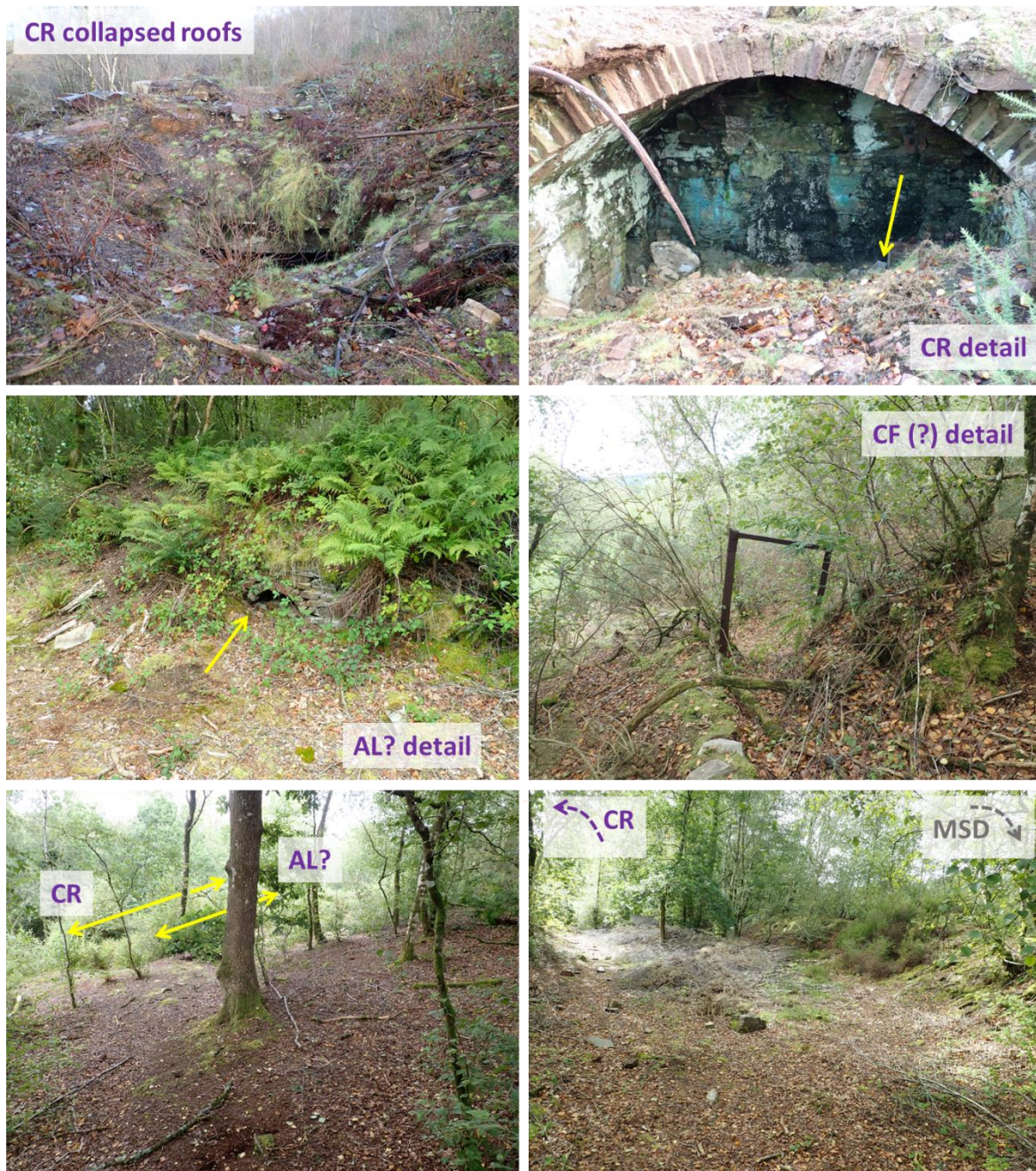
Figure 6-2 Appearance of the area around the calciner row (CR). Top row: the collapsed line of roofs is photographed looking east. CR detail: easternmost calciner, showing a sharp metal spike, efflorescent salts, rubble and a food container (arrow) on the ground (also see Figure 3-5, Figure 4-2 and Figure 4-3). Middle row: partially buried ruined building with arched openings on higher ground south of CR, with remains of channels and iron gates, potentially the calciner flue (CF?) leading to the arsenic labyrinth (AL?). Bottom row: area above CR and AL? (orientation marked by yellow arrows) accessible by site entrance C and level ground between CR and MSD. Abbreviations as labelled on map in Figure 6-1. Photos: C Braungardt 2022&23.
