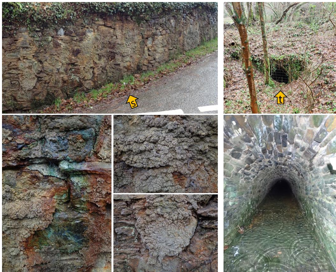
Figure 4-12 Structures associated with the mine site include the Count House (yellow arrow [s] in Figure 4-1), that features a road-facing section of wall upon which efflorescent salts and metal precipitates are evident (left block of photographs). The adit portal is marked [t] in Figure 4-1 and is the entrance to a well-preserved tunnel that runs north, with water flowing south. Photos: C Braungardt 2023.
