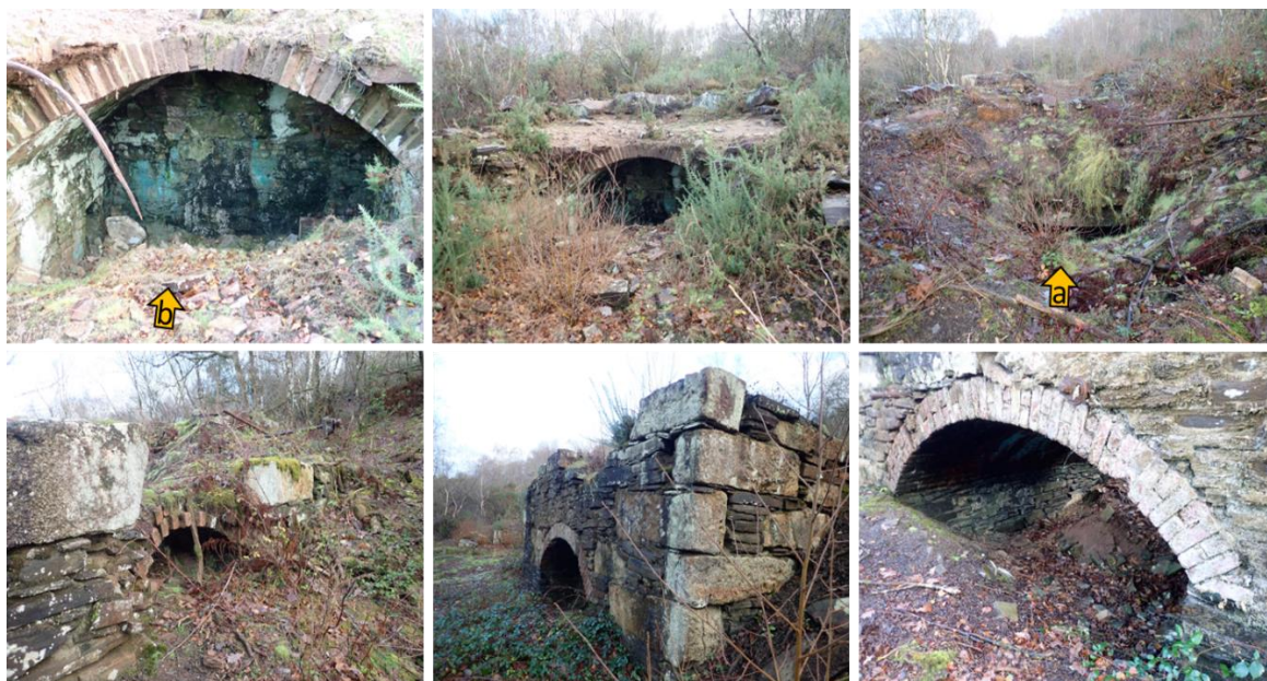
Figure 4-2 Images taken at the row of calciners at NGC, showing individual calciners in various states of repair. The top right image offers a view over the top of the calciner row. Compare with Figure 3-5 from 2005 in Section 3.3. Yellow arrows correspond with viewing angles in Figure 4-1. Photos: C Braungardt 2022.
