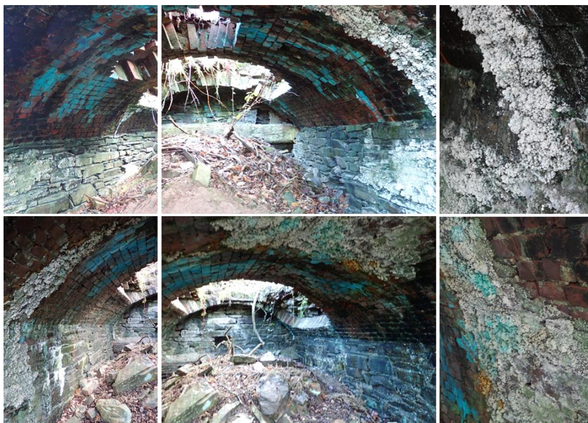
Figure 4-3 Images taken at the row of calciners at NGC in November 2022, showing the inside of two calciners with collapsed roofs, each in a separate row. Detailed photos of the interior show thick, whitish blooms of efflorescent salts and turquoise and ochre metal precipitates on the brickwork. Deposits at the floor of the calciners originate from collapsed roofs and include bricks and mortar impregnated with arsenic, sulfur and metal fumes during calcination and potentially efflorescent salts fallen from the brickwork. Compare with Figure 3-5 from 2005 in Section 3.3. Photos: C Braungardt 2022.
