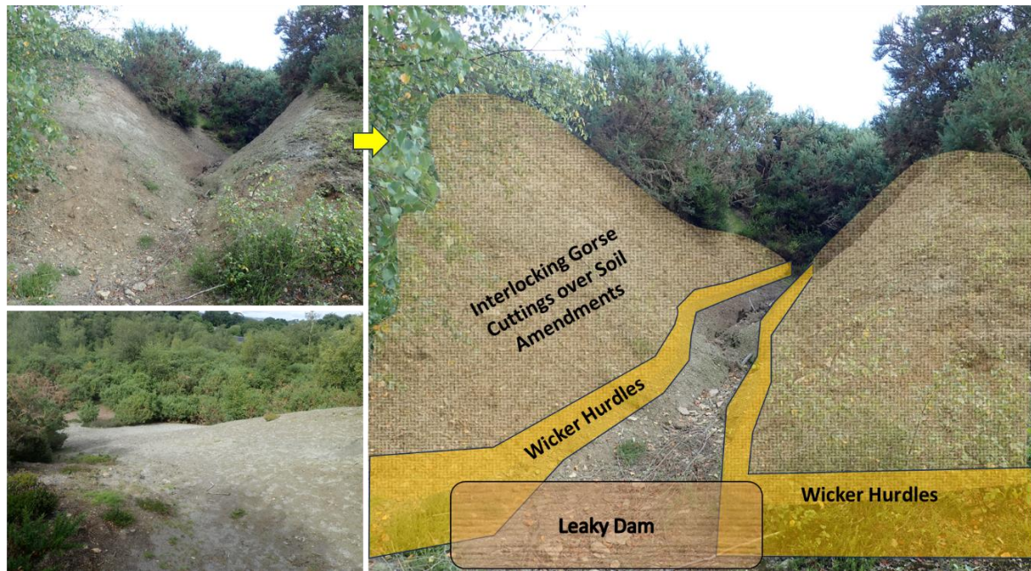
Figure 6-8 Erosion control at slopes using leaky dams and hurdles made from natural materials (willow, hazel) at the base of slopes and drainage points. Interlocking cuttings of brash wood from thorny vegetation, such as gorse, can be used to cover the slope from the base up to hold soil amendments in place. Top left and main image: steep slope 7d in Figure 6-7. Bottom left: moderately steep slope 6 in Figure 6-7.
